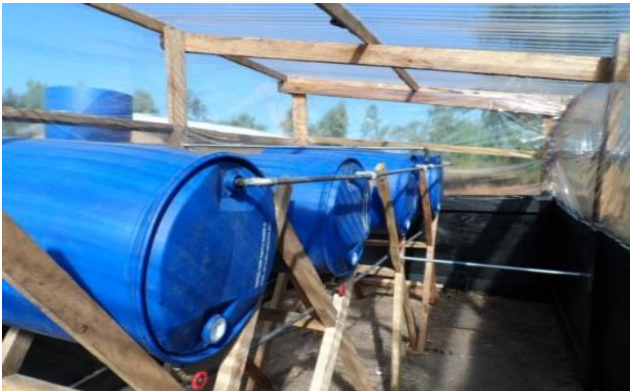
Figure 4- Inside layout of the solar still design at project site
