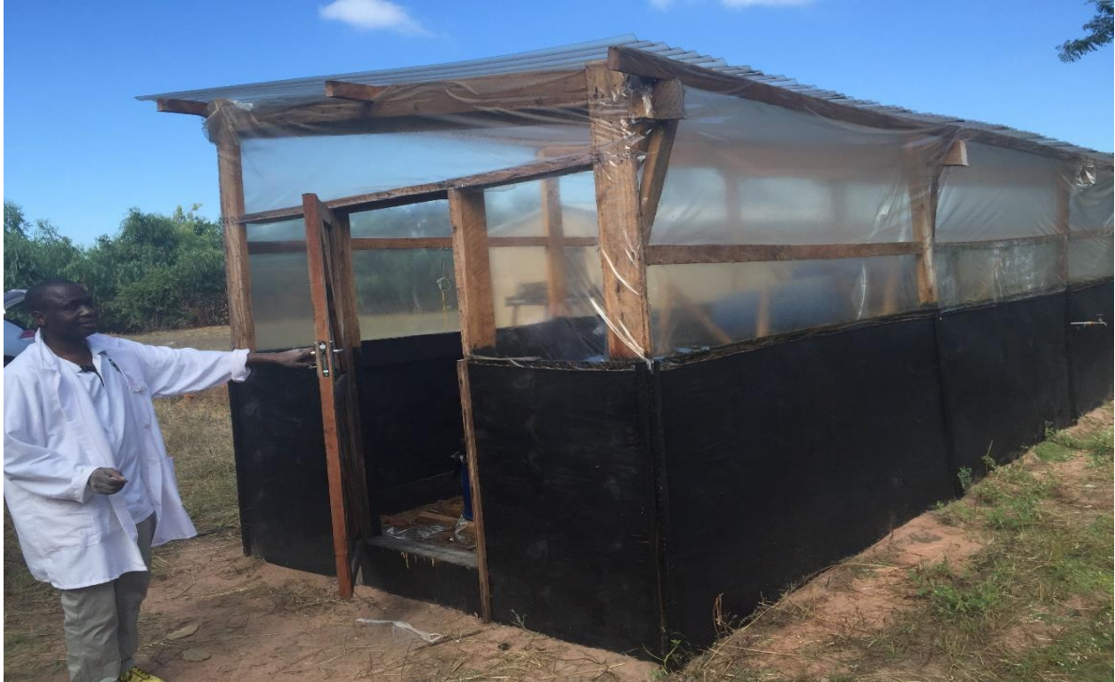
Figure 3- Solar still design at project site
